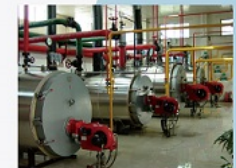
0.7MW Gas Fired Hot Water Boiler in Kazakhstan
