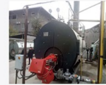
6Ton/h Gas Fired Boiler in Uzbekistan
