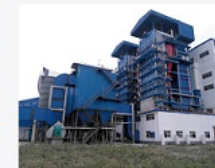
75Ton/h Circulating Fluidized Bed Boiler in Cuba
