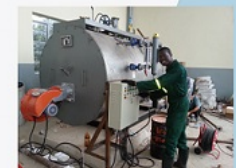
2Ton/h Diesel Fired boiler in Nigeria
